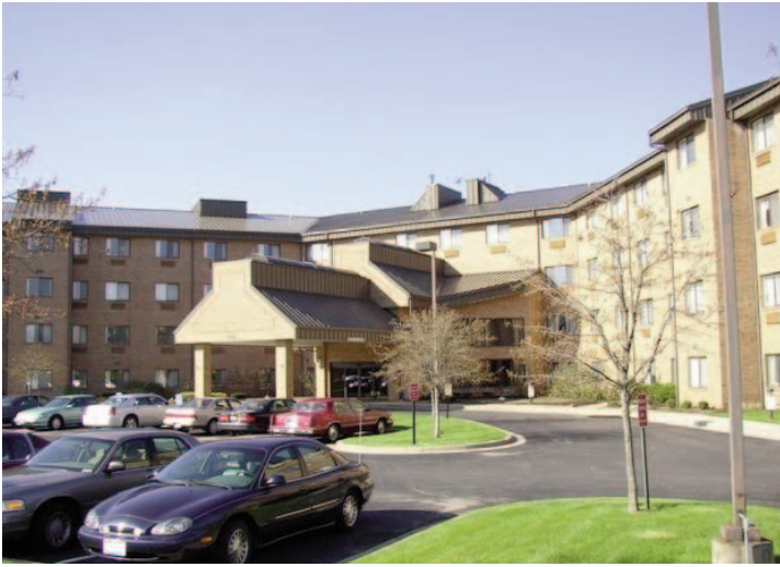
Sycamore Glen Retirement, Miamisburg, Ohio New standing seam metal roof system after existing metal roof was removed.
